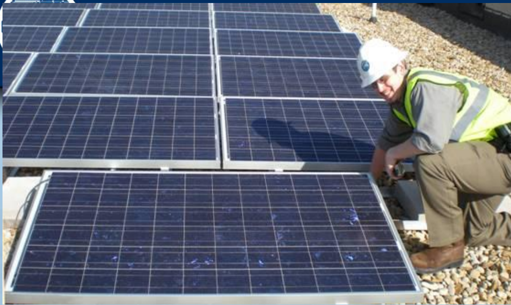
Photovoltaic System Construction and Installation, Buildings 1050 and 2155, Hickam AFB, Hawaii
